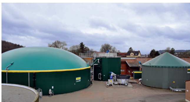
New biogas research plant at HBFZ for power supply in line with demand
