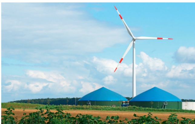
Biogas plants play a vital role in demand-oriented electricity generation (Photo: fotalia.com).
